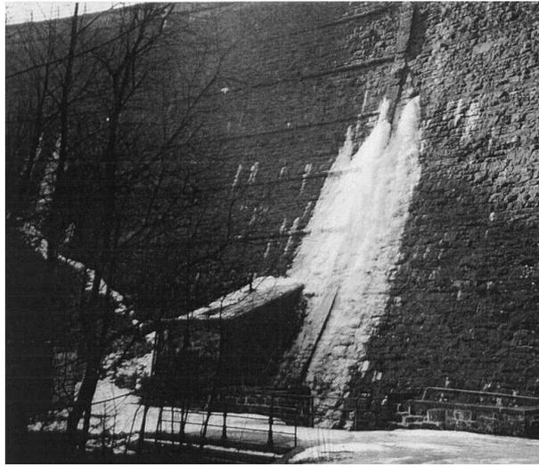
Figure 1. Frozen seepage water along the downstream side of a dam (Source: Ruhrverband, Essen, Germany). Undesired percolation is a common indicator for local damages.
